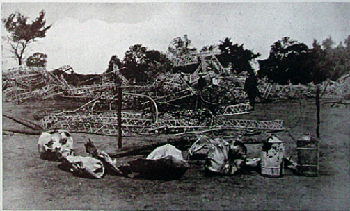
PETROL TANKS AND SUPPLY CANS.
